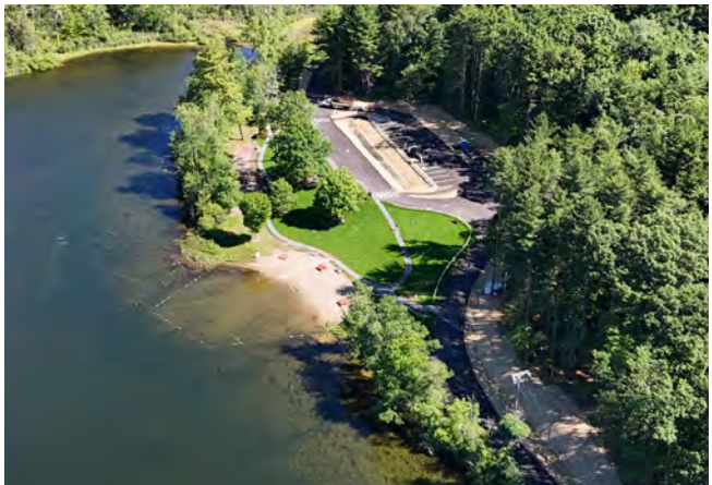
Years of improvements to the Lake Mansfield Recreational Area are nearly complete. The road has been moved farther from the beach area and measures have been taken to mitigate traffic and runoff into the lake, making it a cleaner and more accessible recreation area. Ben Garver, The Berkshire Eagle, Friday, June 28, 2024.
