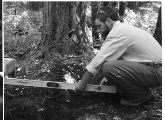
Peter Jensen directs bridge construction
