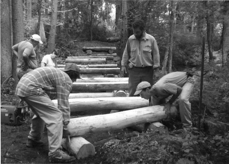
Volunteers place bridge footings
