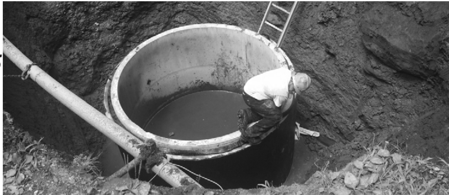
One of the newly installed catch basins on Castle Hill Avenue.
