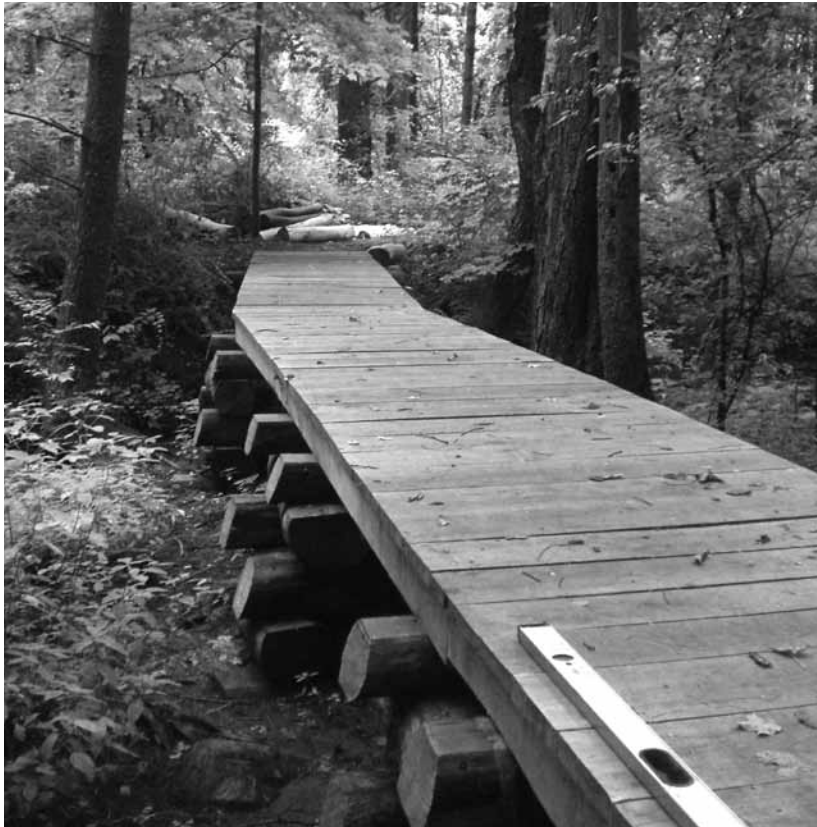
A bridge/boardwalk provides passage through a sensitive habitat area
