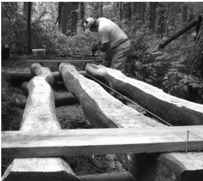
Bridge decking is mounted on stringers
