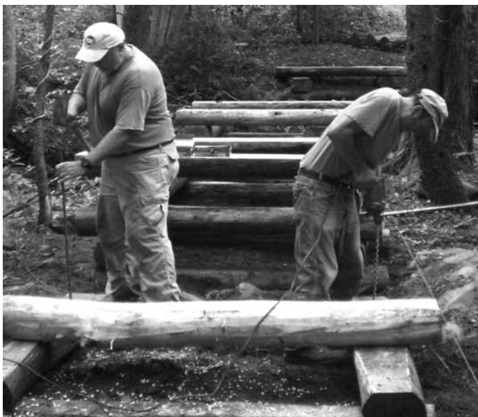
Ron and George set footings
